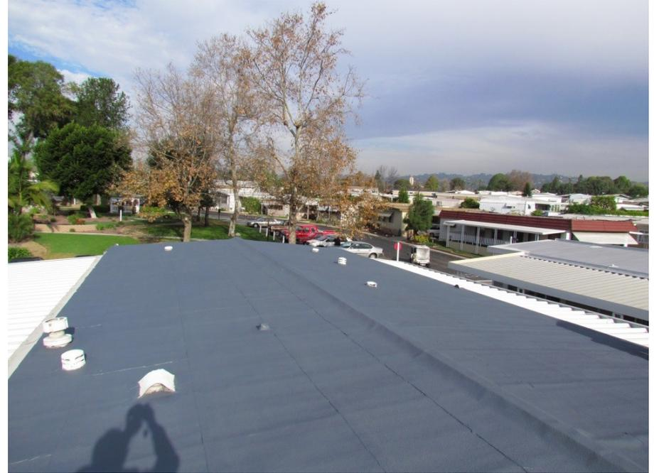
The Rubber coating is designed to be a water-resistant, protectant surface, that provides extra sound absorption for your roof.
